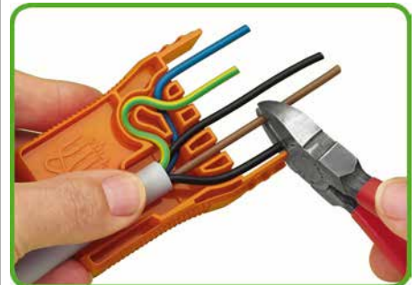
Cut conductor ends.
