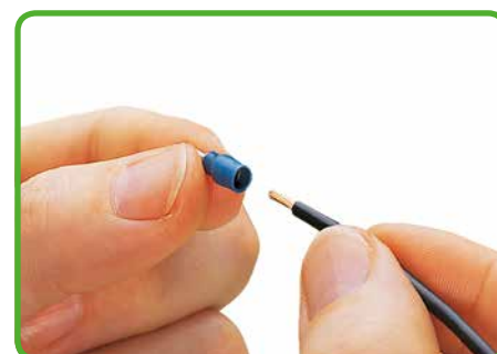
Push the pin terminal onto the conductor.
