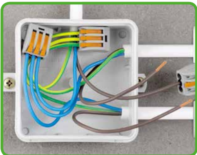
Wiring fine-stranded conductors in a junction box.
