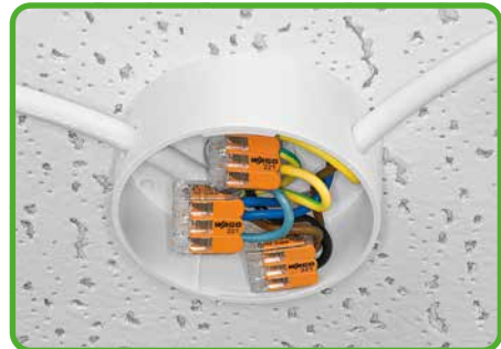
Lighting distribution in ceiling canopy
