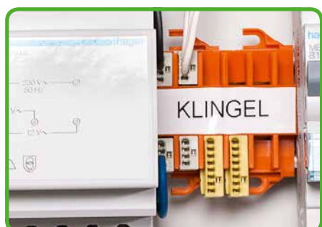
Example of residential door bell application - mounted on DIN 35 rail
