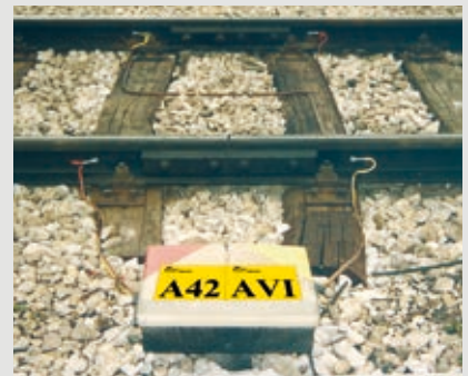
Rail circuit box
