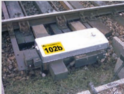
Switch shunting box
