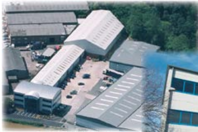
Cembre Ltd. factory in Curdworth (Birmingham)
